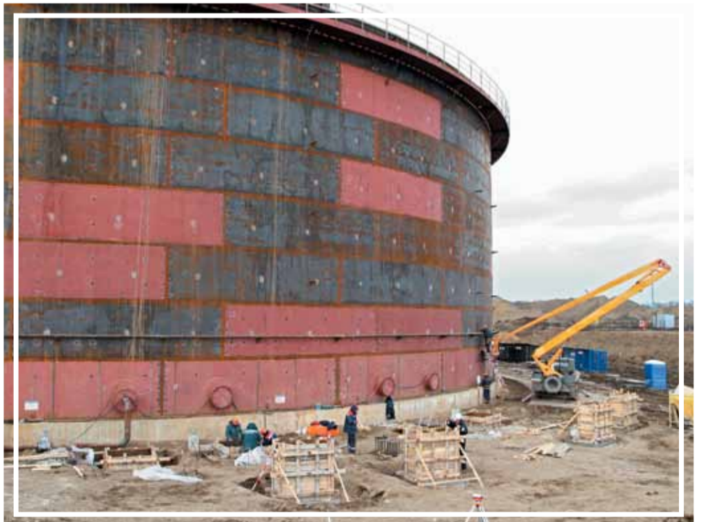
Arrangement of foundations for pipe headers at Kropotkinskaya PS
