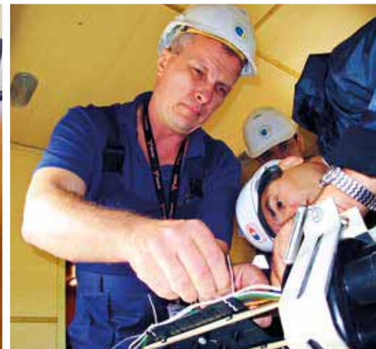
Fiber-optic coupling installation
