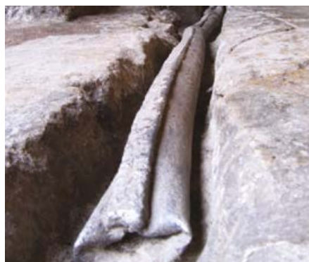
Sometimes during excavations we find metal pipes with channeled edge bents packed with sealant. However, to preserve their air-tightness they had to be embedded into the masonry constructions
