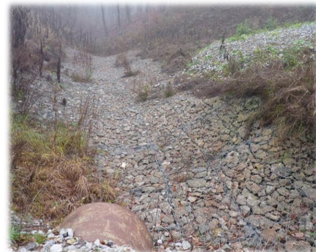
Temporary stream reinforced with Reno mattresses
