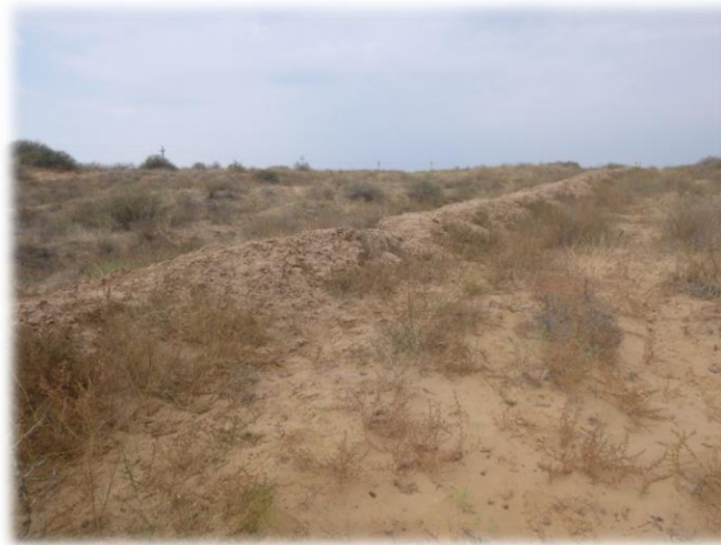
Soil recently filled over the pipeline route to prevent the fine soil wind erosion and comply with the pipeline process depth.
