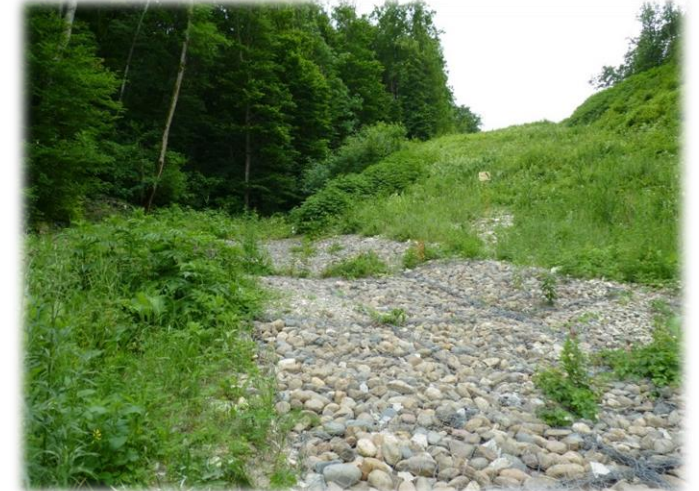
Land slide hazardous area reinforced with Reno mattresses
