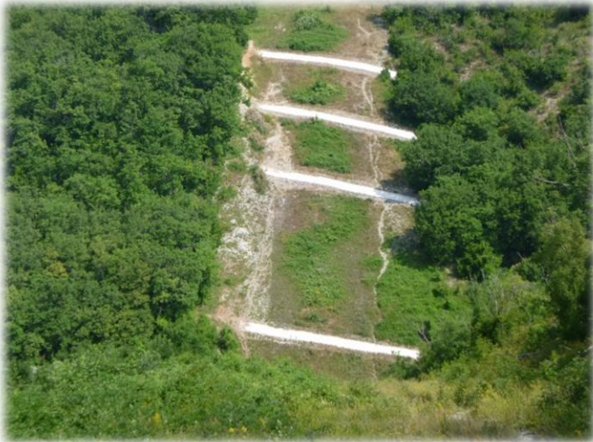
Protective barriers to prevent erosion
