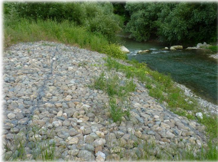
Reno mattress reinforced bank at the pipeline Bakanka River crossing
