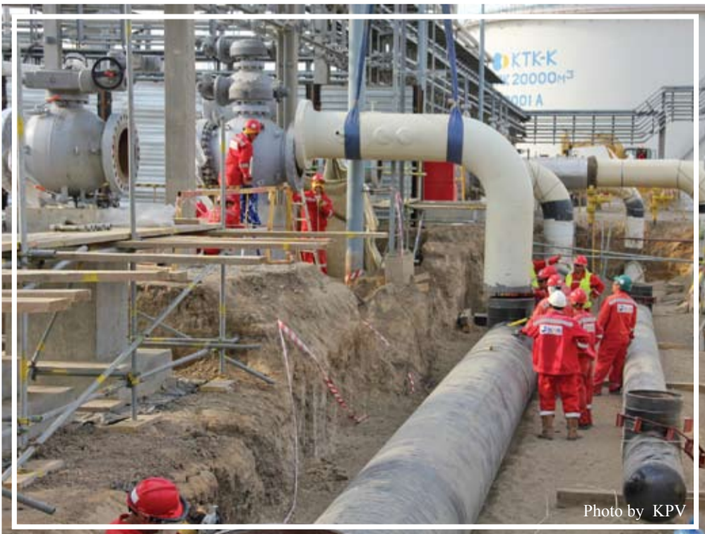
Mainline pump piping installation, Atyrau PS
