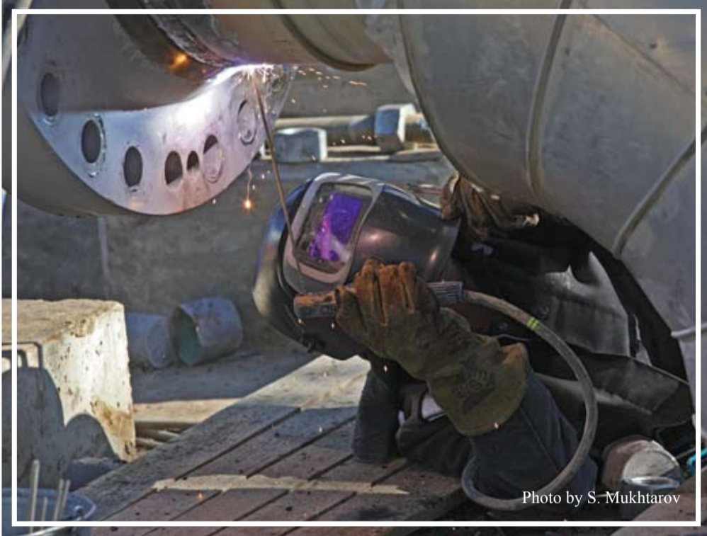
Welding during ball valve replacement, Kropotkin PS
