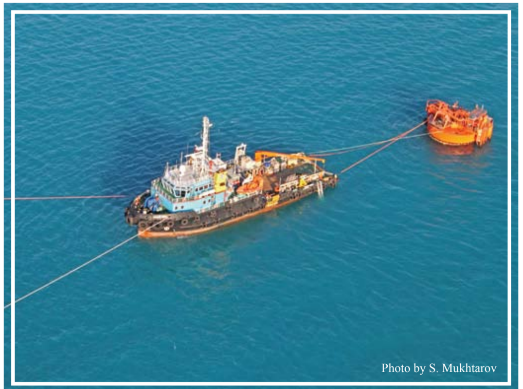
SPM hose replacement, Marine Terminal offshore area
