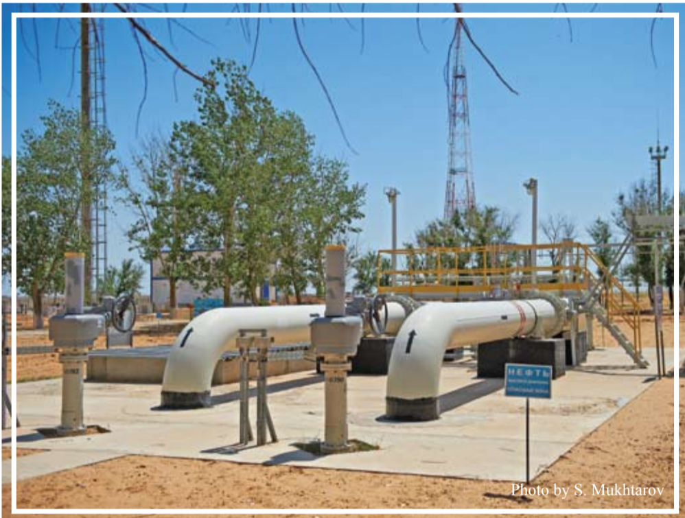
Outlet pressure control station, Astrakhan PS
