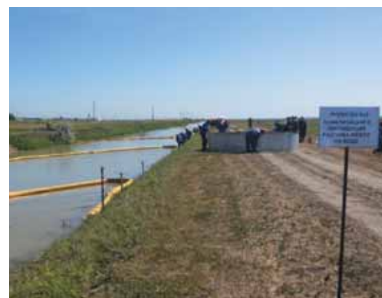
Deployment of containment booms and installation of a temporary storage tank
