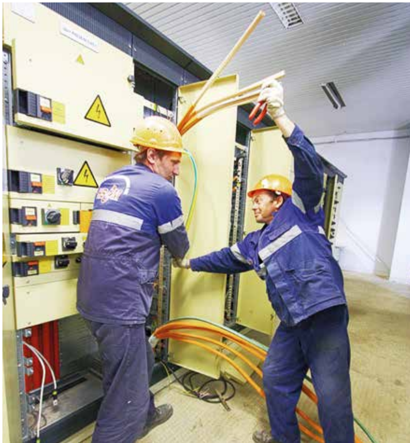
Each control cabinet accommodates 38 cables
