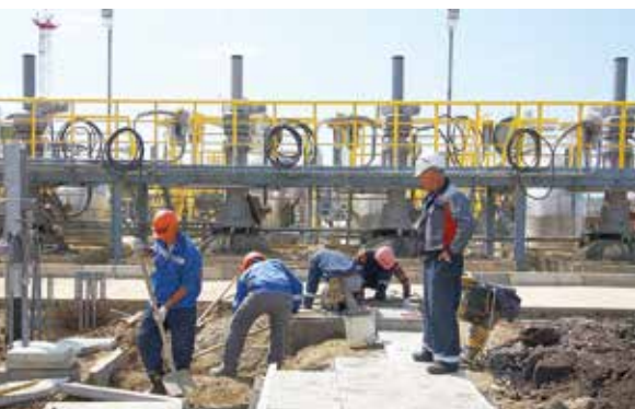
Site improvement. Construction of a walkway to mud strainer units
