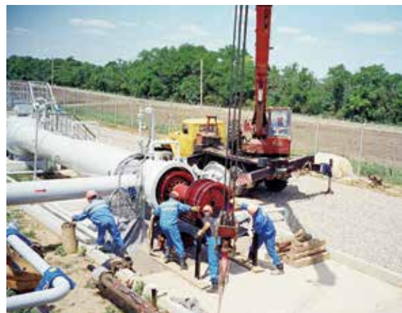
The kicking of an “intelligent pig” into a pipeline is not an easy thing to do
