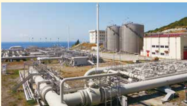
From the tank farm, oil flows by gravity to the shore facilities
