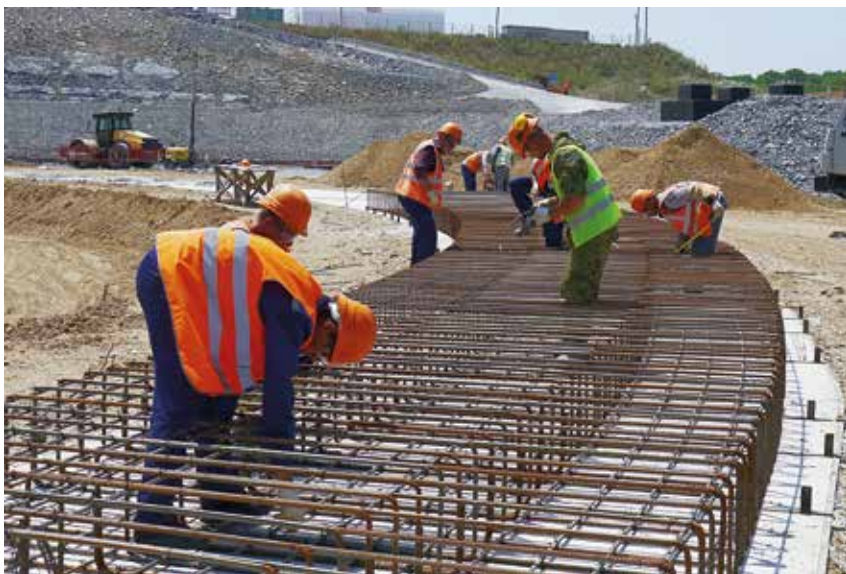
Tank foundation reinforcement
