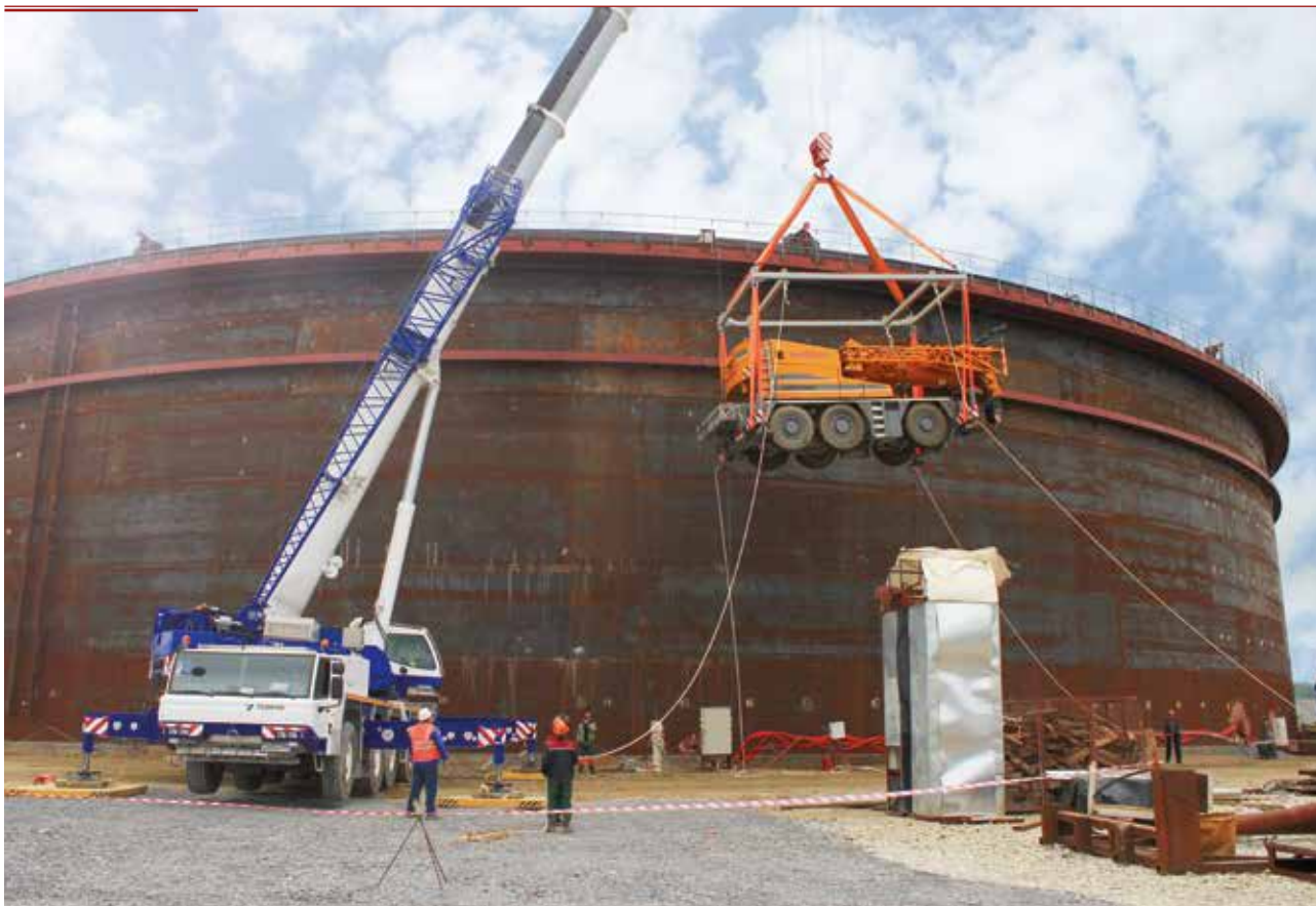
This was the first such operation to be carried out in Russia to remove cranes from 100,000 m 3 tanks with a wall height in excess of 20 m.
