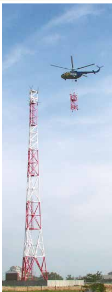
Installation of a radio-relay tower at PS "Kropotkinskaya" (Russia)
