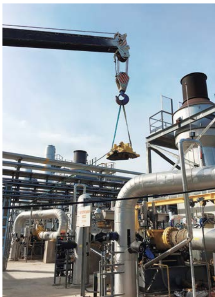
Fitting the mainline pump cover
