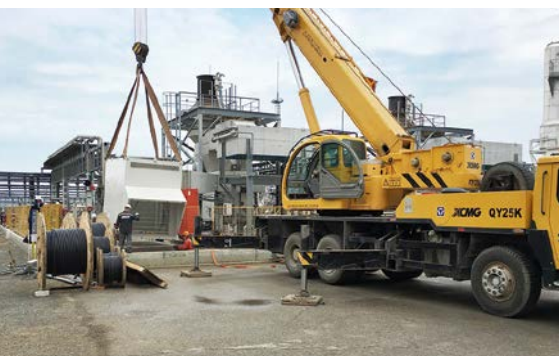
Installing the oil cooler enclosure
