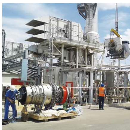
Dismantling of the existing turbine and preparation for installation of the new one
