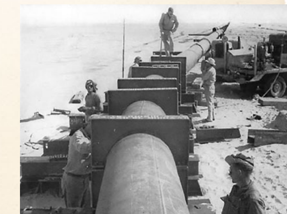
In Saudi Arabia, the oil pipeline section was mounted on special supports
