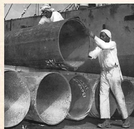
When transporting by ship, small-diameter pipes were placed into large diameter pipes
