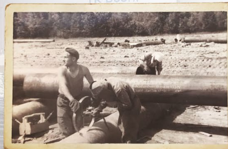
Pipe-welding station. Laying pipelines. 1960s. Aktyubinsk Region
