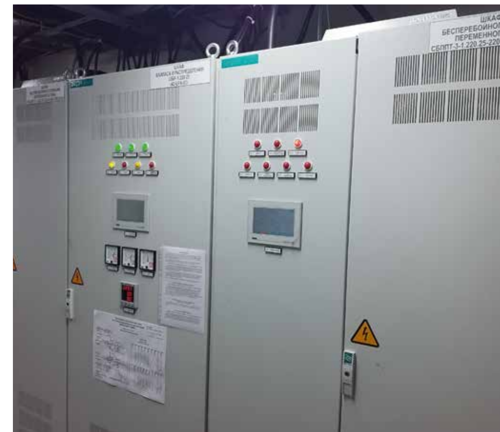
MARINE TERMINAL TANK FARM. GENERAL VIEW OF UNINTERRUPTIBLE POWER SUPPLY UNIT (UPS)
