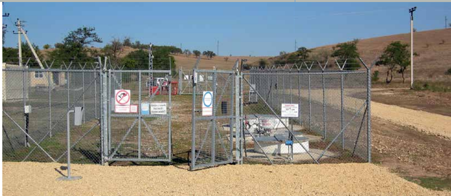
A BLOCK VALVE STATION IN THE LINEAR PORTION
