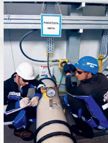
MAINTENANCE OF THE BOLID FIRE DETECTION SYSTEM AT A-OPS 4A
