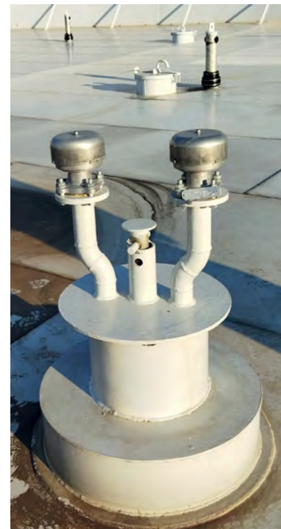
UPGRADED AUTOMATIC DISCHARGE VALVE SVFRT-100000
