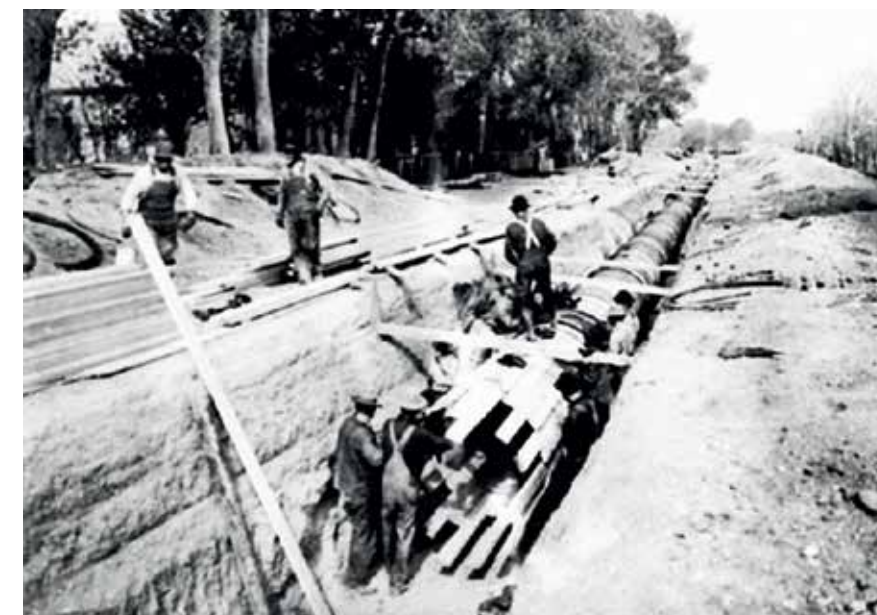
LAYING A 48-INCH WOODEN PIPELINE IN DENVER, COLORADO, 1910
