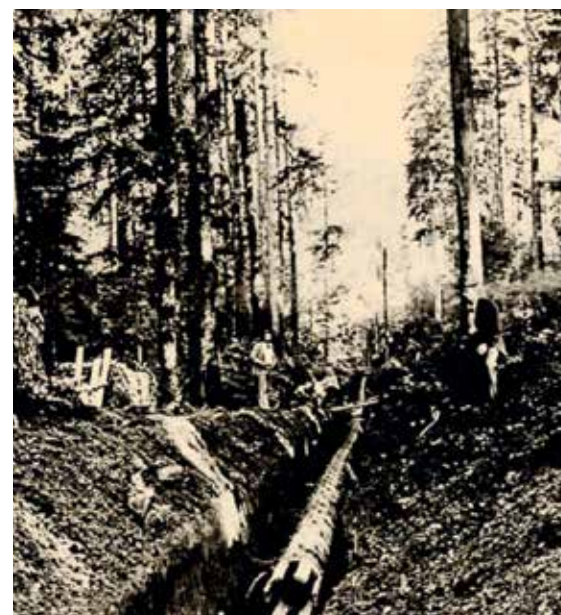
LAYING A WOODEN PIPELINE NEAR ASTORIA, OREGON, 1884
