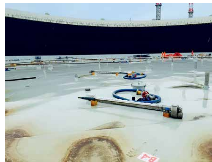
PREPARING FOR WASHOUT. IN THE FOREGROUND IS A ROTARY EROSION HEAD
