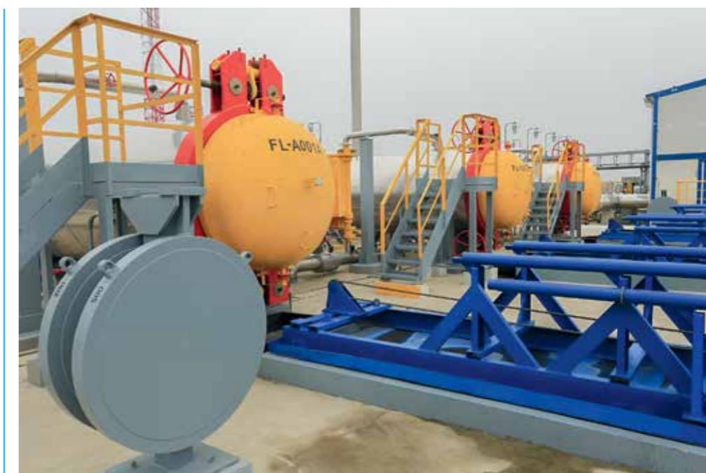
SAFETY FENCES AT THE SITE OF PS-8
