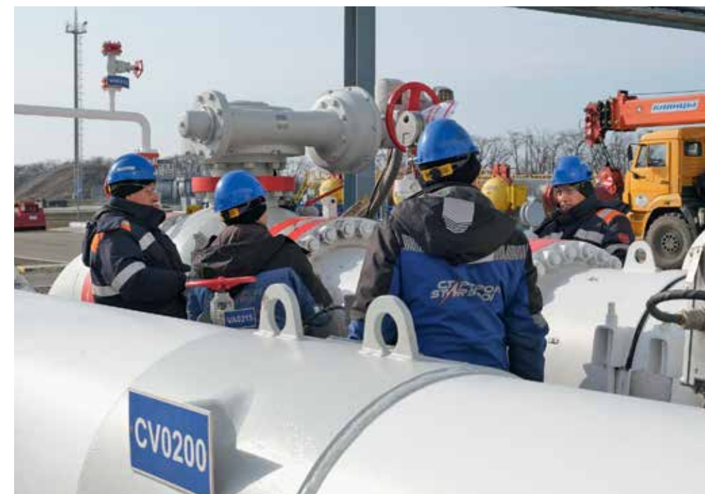
CONTRACTORS PERFORM DOUBLE SEALING OF THE STATION'S PROCESS PIPELINES
