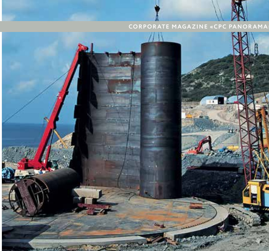
ROLLED INSTALLATION OF A 9500 M 3 TANK
